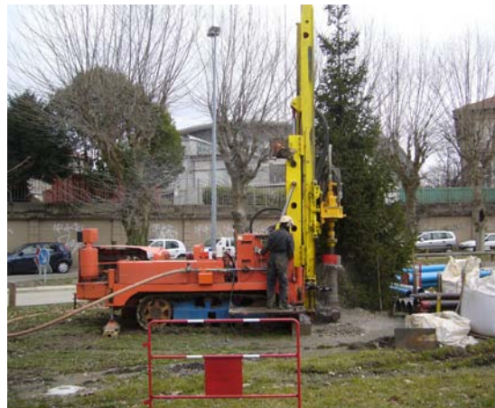
Drilling of a test borehole
