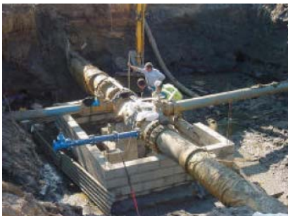
Pressure network 90 km long - 100 to 600 mm dia. - NP 25 bar
