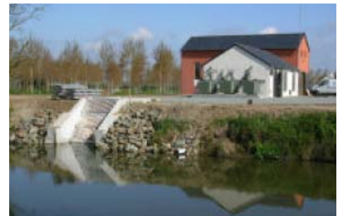
Pumping station on the Authion Discharge: 3600 m 3 /h Delivery height: 165 m
