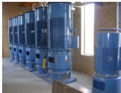
Pumping station on the Authion Discharge: 3600 m 3 /h Delivery height: 165 m
