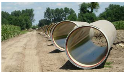
Loire – Authion feeder pipe 3000 m long - 1200 mm dia. FRP
